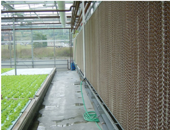
Evaporative cooling pad used to lower the greenhouse temperature when the ventilation system alone is not sufficient to maintain the set point temperature.
