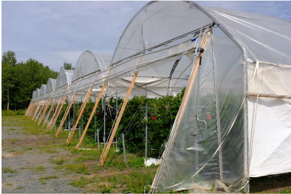
Figure 4. End wall design for raspberry production in gutter-connected high tunnels.
