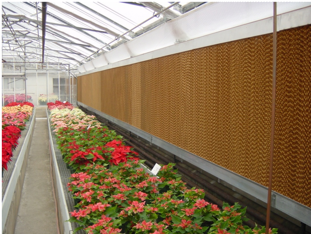
Figure 1. Evaporative cooling pad installed along the inside of the ventilation inlet opening.
