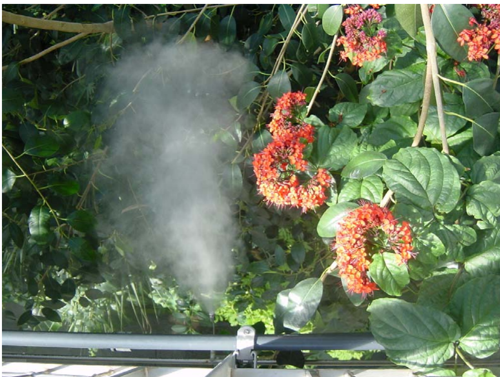
Figure 2. Top-down view of a fog nozzle delivering a small-droplet mist for evaporative cooling.
