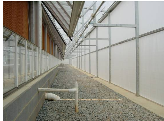
Picture 5. Partially opened side wall ventilation window showing an externally installed insect screen on the right and an internally installed evaporative cooling pad on the left.
