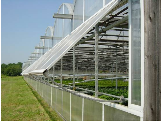
Picture 1. Fully opened side wall ventilation window in a mechanically ventilated greenhouse.
