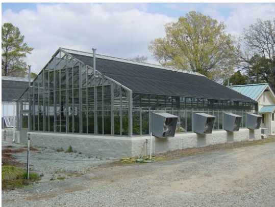
Picture 3. Mechanically ventilated greenhouse with an external shade curtain.
