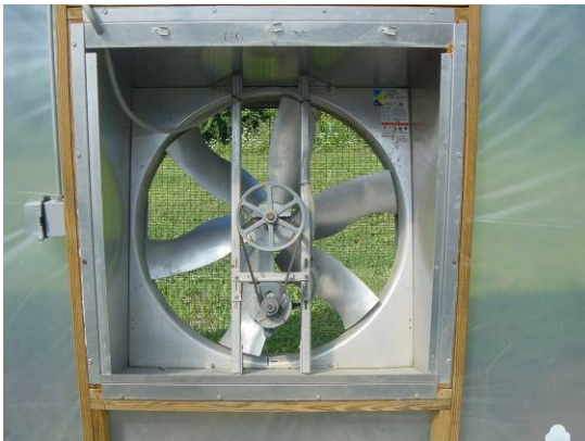
Picture 2. Exhaust fan shown from inside the greenhouse with the louvers removed.
