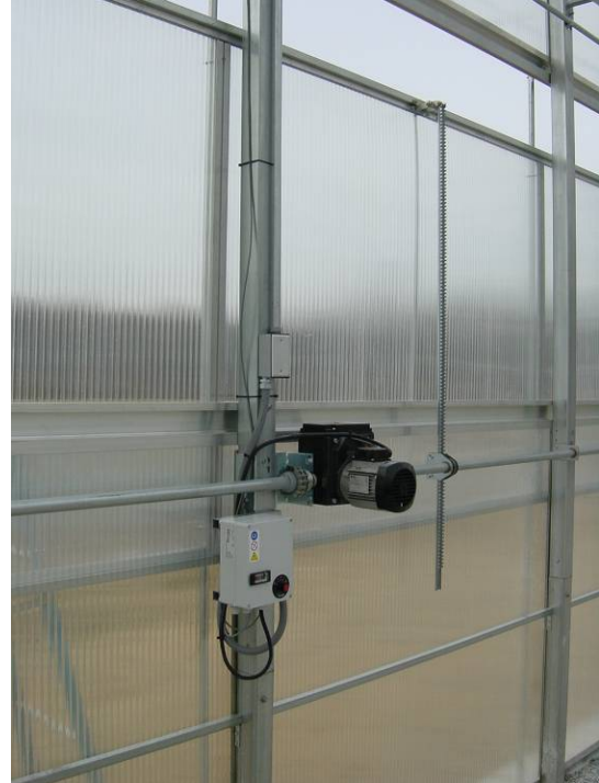
Picture 4. Drive motor and gear box for a vertically operated side wall ventilation window.
